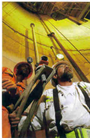
Shaft Sinkers personnel at Lonmin Platinum's Saffy Shaft.
